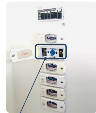
N 2 O pipeline supply switched off in NUH Medical Centre OT
